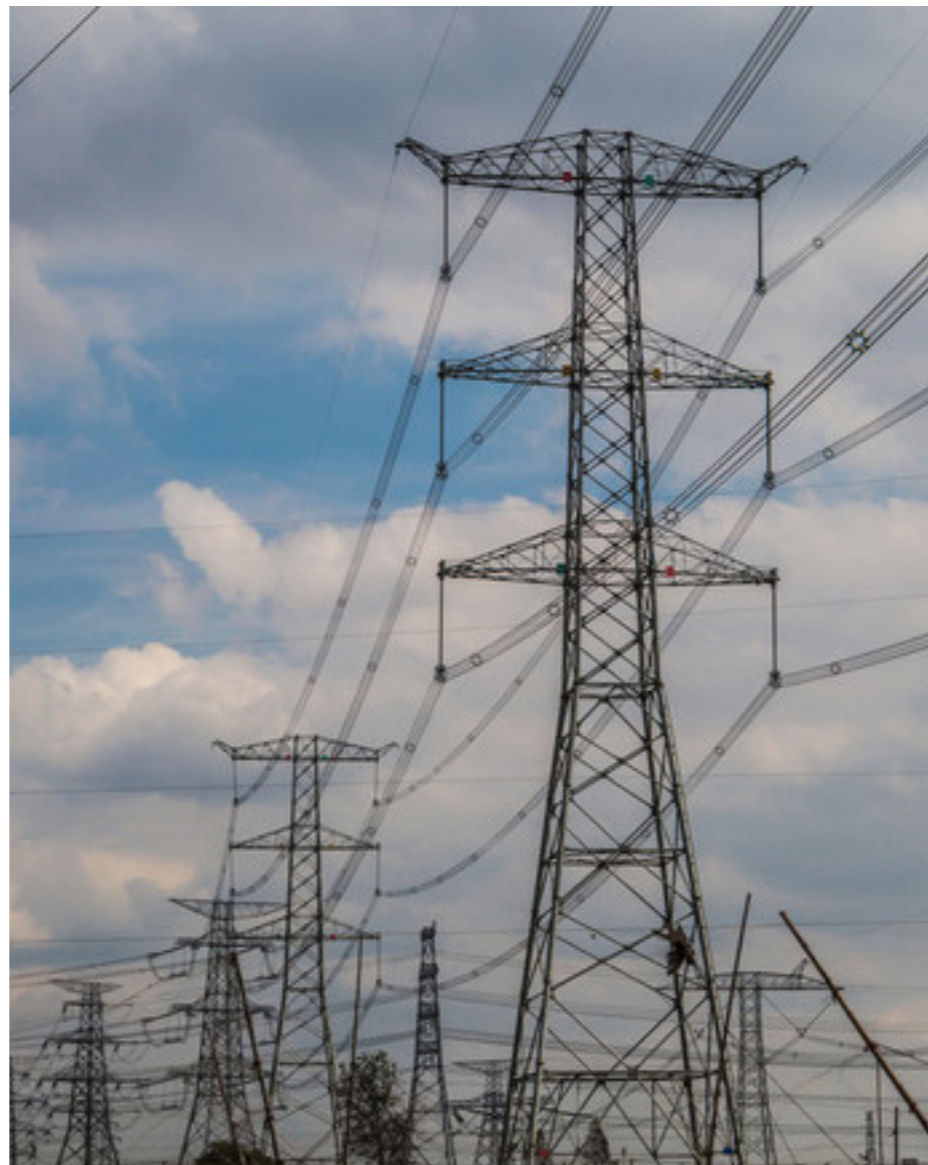
基地内高压电塔密集穿越 ELECTRICITY PYLONS PASSING THROUGH THE SITE
