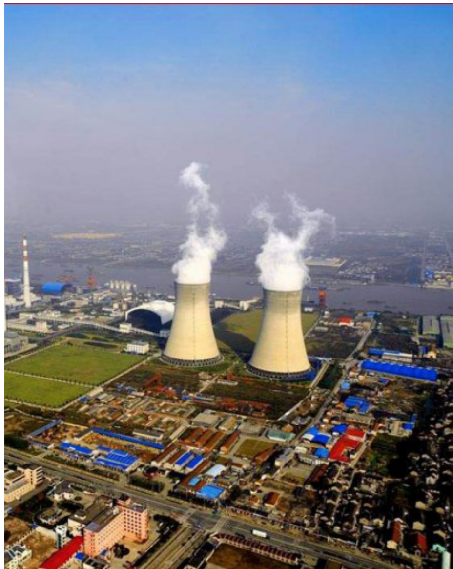
上海吴泾第二发电厂,化工厂等离基地两公里 POWER STATION, CHEMICAL PLANT NEARBY 2KM
