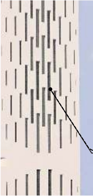
Residential facade frame - lower parcel Window wall system with metal screen. Apperance of punched window wall.
